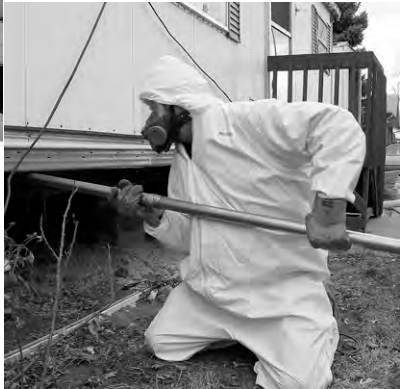
Patching a flexible belly: The technician uses both adhesive and stitch staples to fasten a patch.
