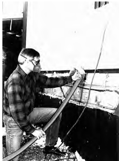
Adding insulation to mobile-home walls: A contractor uses a fill tube to install more insulation in a partially insulated mobile-home wall.
