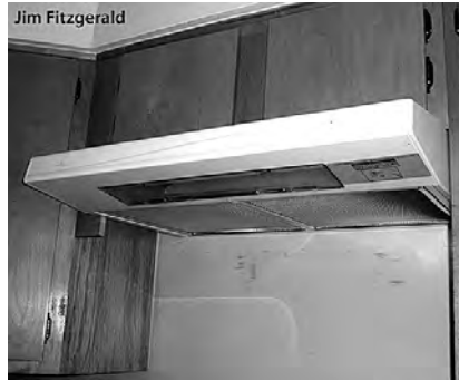
Advanced 4-speed range fan: Lower speeds for continuous ventilation and higher ones for spot ventilation.
