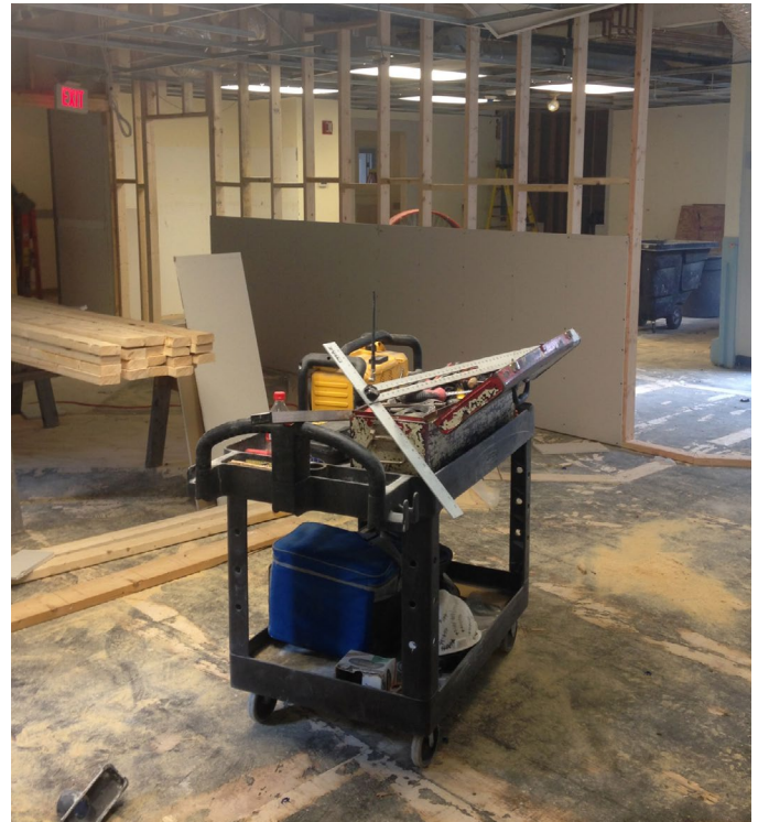
Classroom Interior - During Construction
