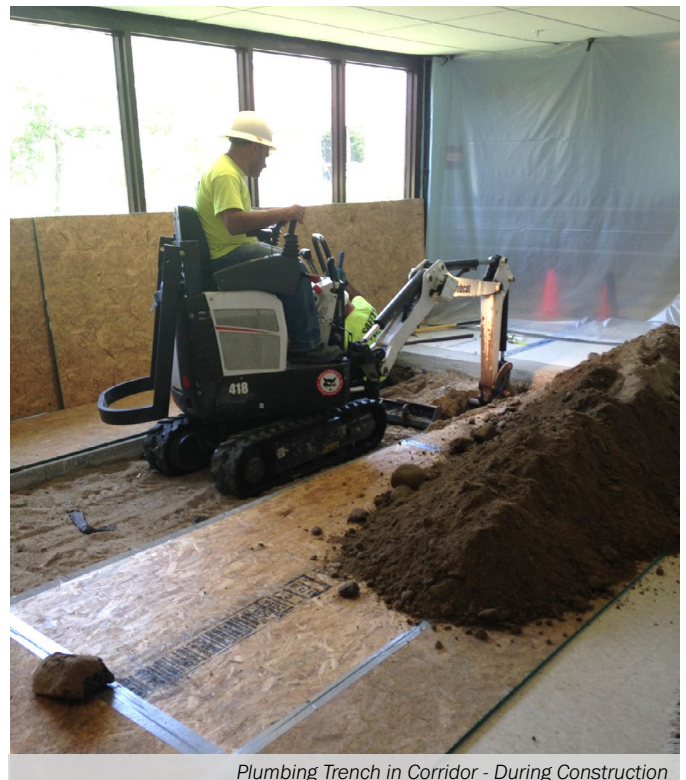
Plumbing Trench in Corridor - During Construction
